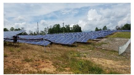
Example of a fixed tilt installation in Conyers, GA on solid rock with ground screw foundations
